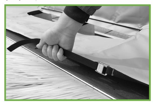
Step 9: push the remaining strap back in the sleeve.
